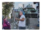
During final renovations to The Turrets, COA's Director of Buildings and Grounds, Millard Dority, led guests up on the scaffolding for up-close Hard Hat Tours. COA replaced 99 windows, over 20 doors, 7 chimneys, and the slate roof. In addition, the entire exterior of the building was repointed.
