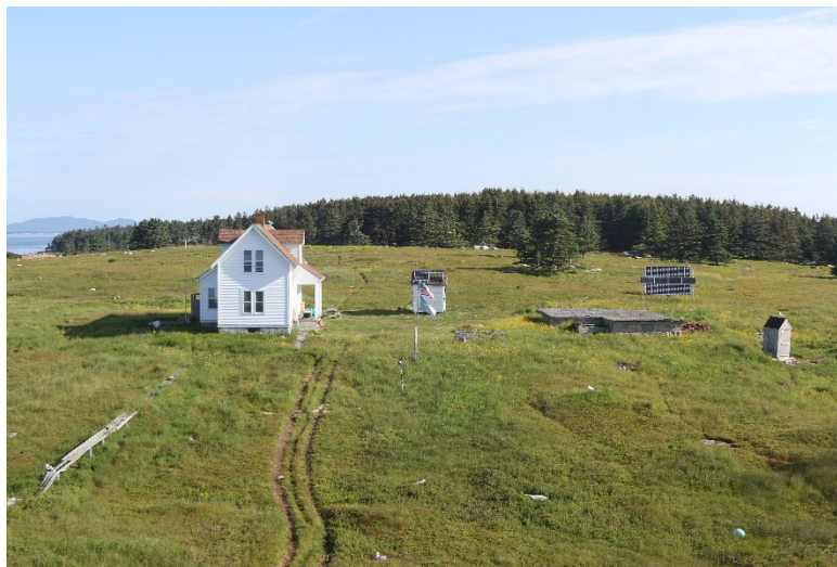
The keeper's house, showing photovoltaic panels (upper right)
