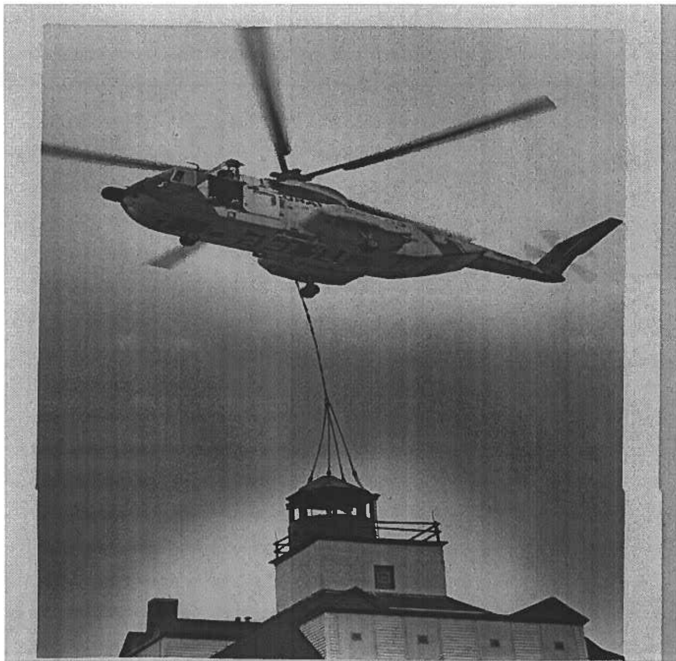
Figure 5 Replacement of the lanternhouse. Courtesy of the Bar Harbor Times
